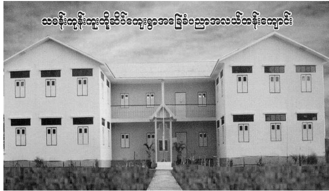
The school is a two storey building measuring 150' x 40', which will accommodate 500 children. Project sponsored by Mr Aye Myint
