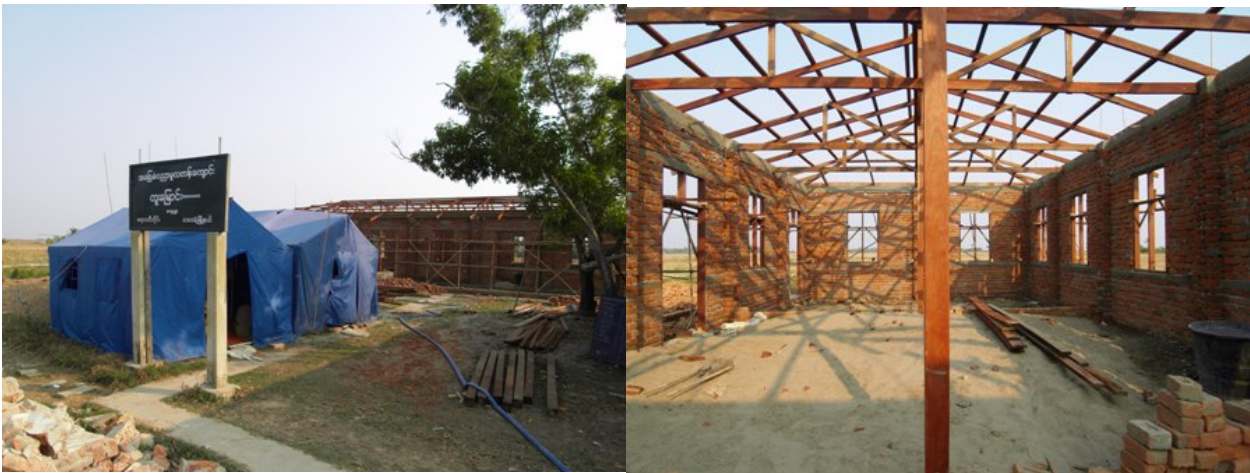
New school under construction at Too-myaun village
