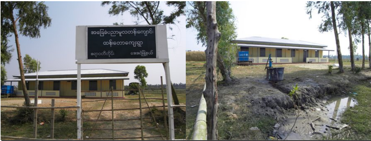
New Primary School at Htan Taw village
